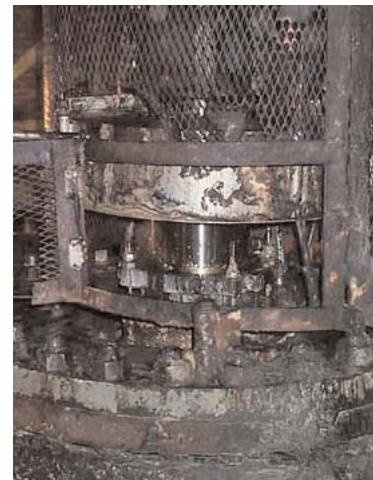
Close-up of Blow Tank - SXL Application
