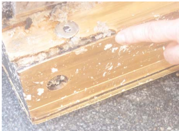
Damaged Brass Wear Strip on Double Press Grinder
