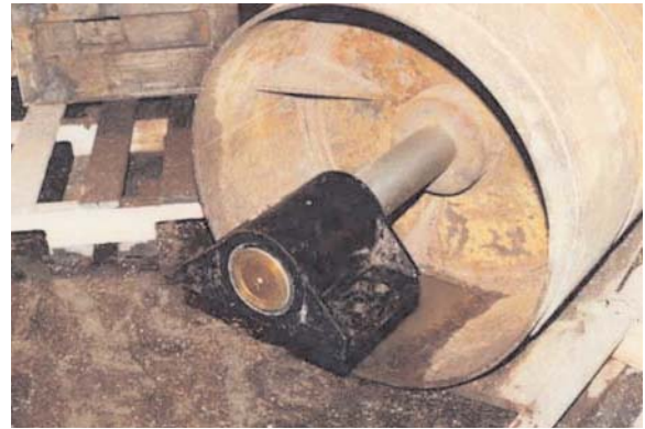
AFTER - Jack Ladder Drum and SXL Pillow Block Bearing Installed
