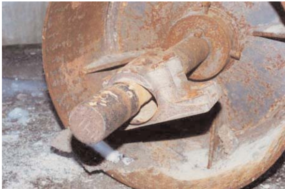
BEFORE - Jack Ladder Drum and Bearing
